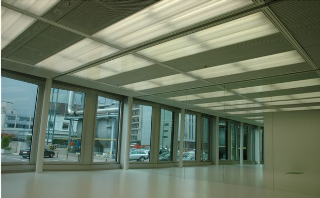
Campus Novartis, Basel: Stretch-metal-ceiling with high-absorption lighting
