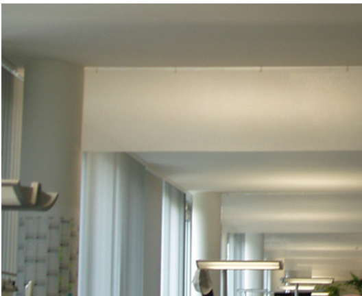
Lining acoustic baffles up over workplaces. The pursuit of transparency and good acoustics do not have to be mutually exclusive.
