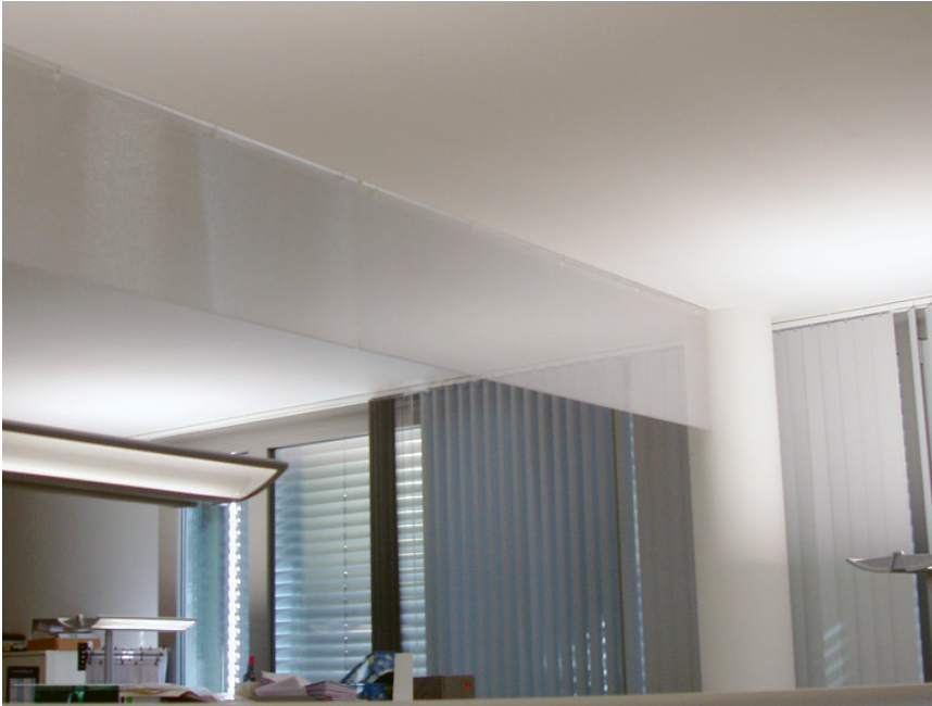
The current trend in contemporary architecture is for ever more transparency, acoustic baffle
